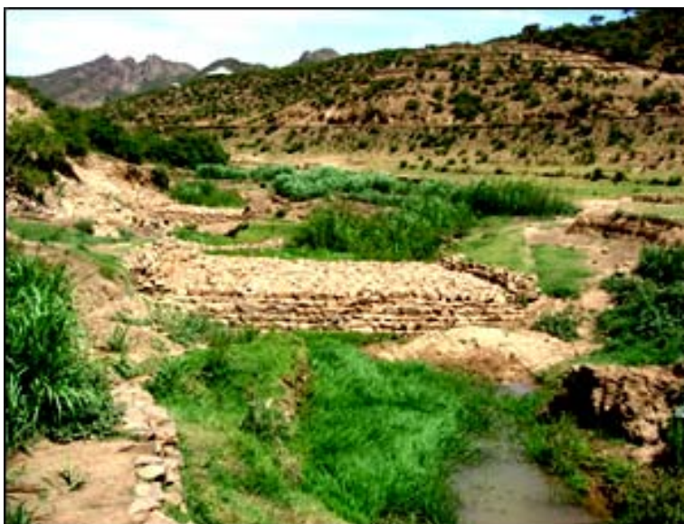
Figure (x): Integration of Check-Dam with Plantation
