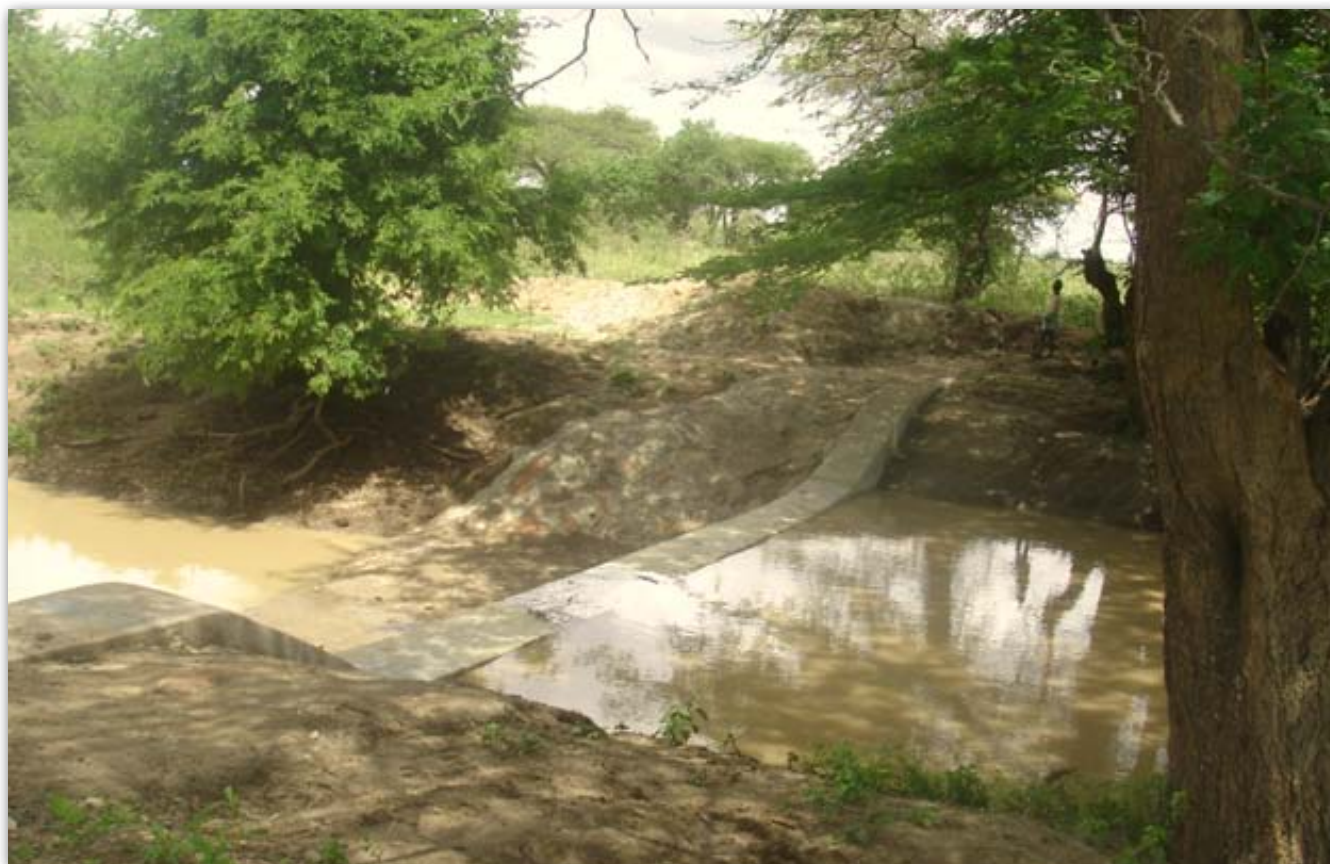
Fig 13.2 Typical masonry sediment storage dam (Kotido)
