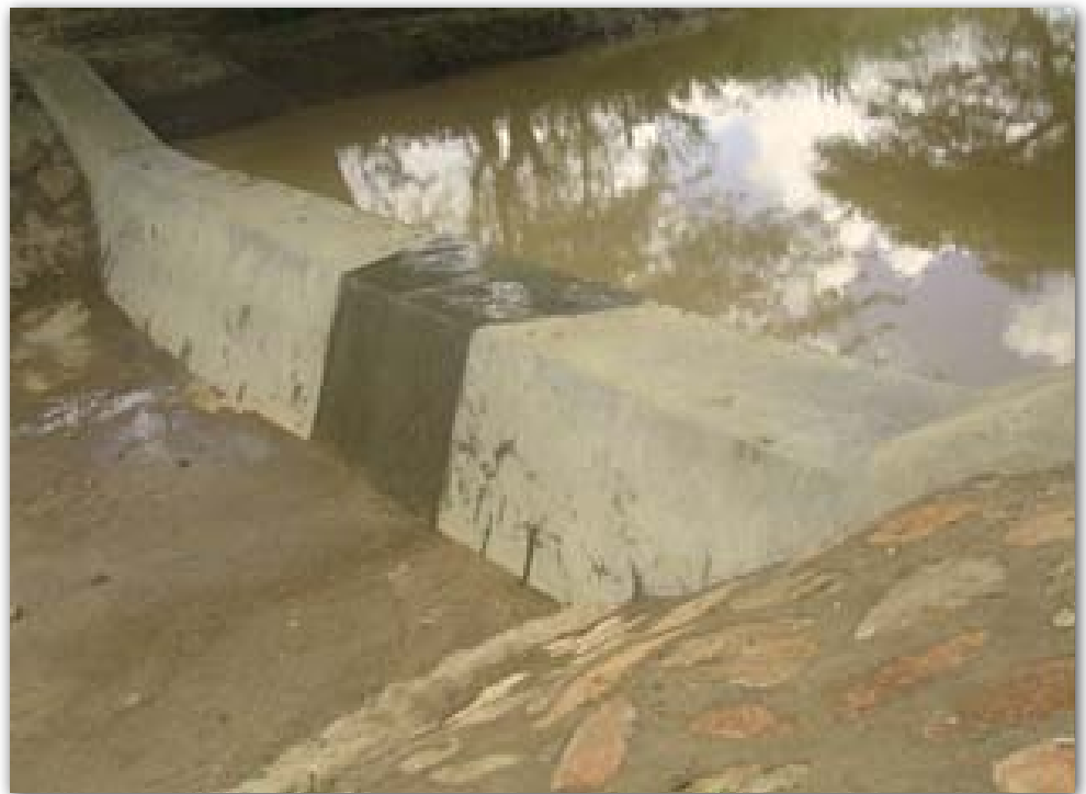
Fig 14.3 Good overflow spillway masonry dam
