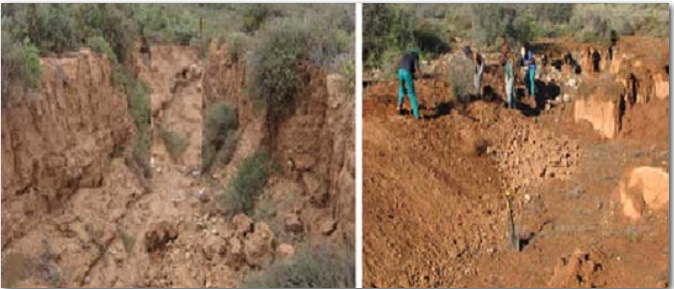
Fig 2.6 Reshaping vertical and deep gully
