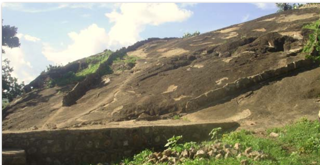
Fig 5.2 Effective runoff water collection rock catchment in Kotido
