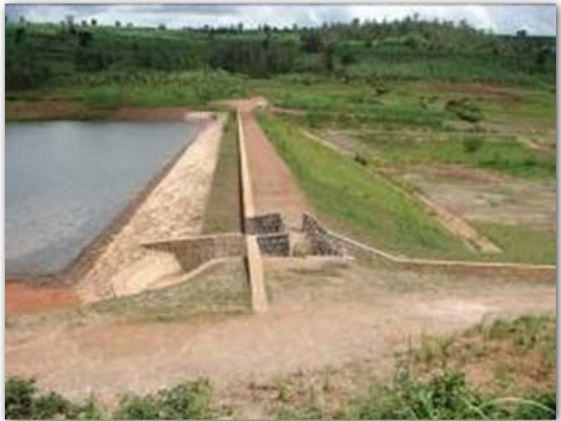
Fig 12.1 Typical view of zoned earth embankment dam
