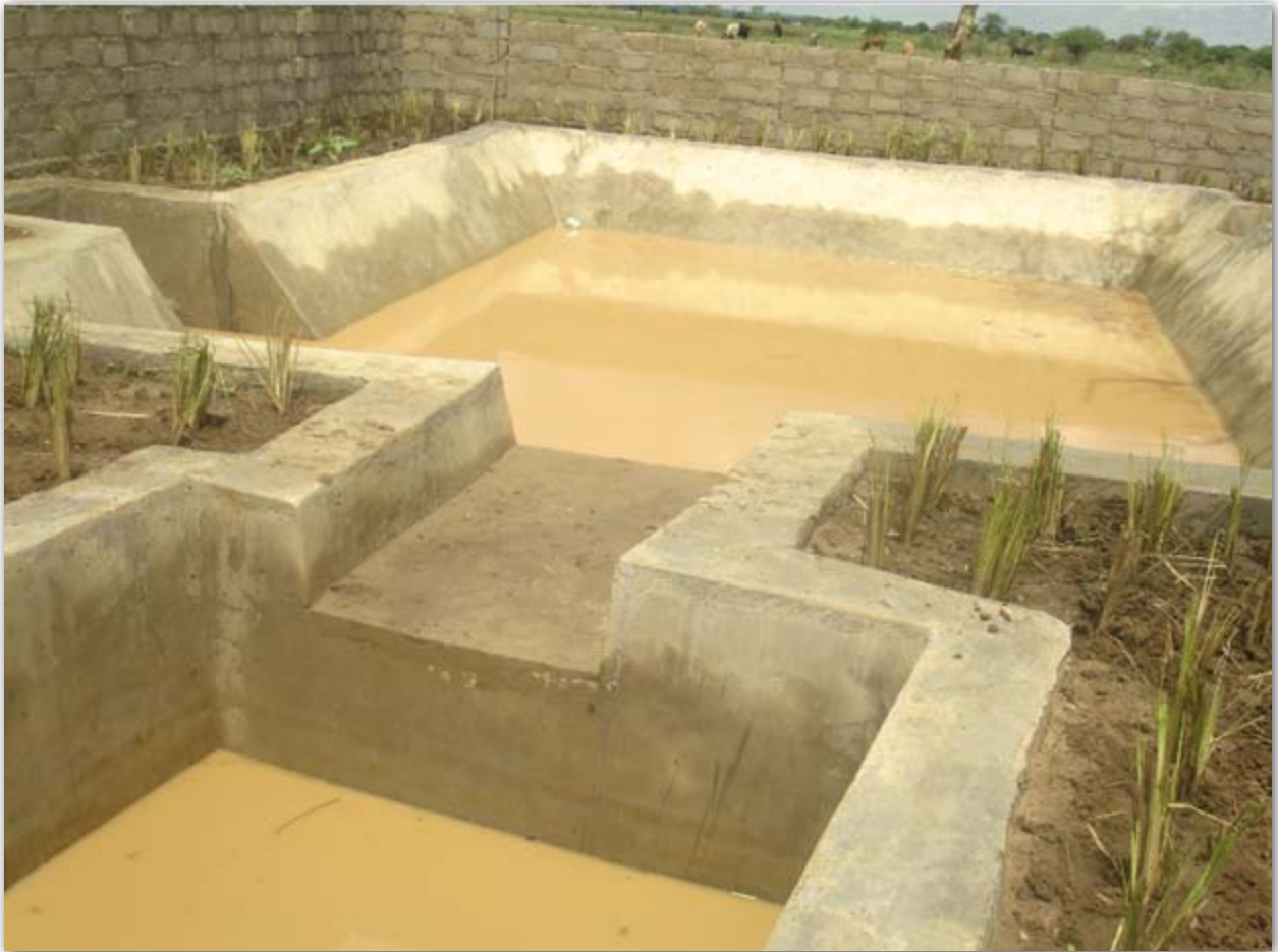
Fig 11.1 Improved design and construction of runoff water harvesting pond (Kotido)
