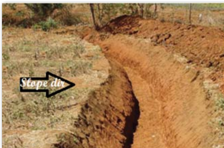
Fig 6.2 Deep water harvesting contour trench for moisture stress areas
