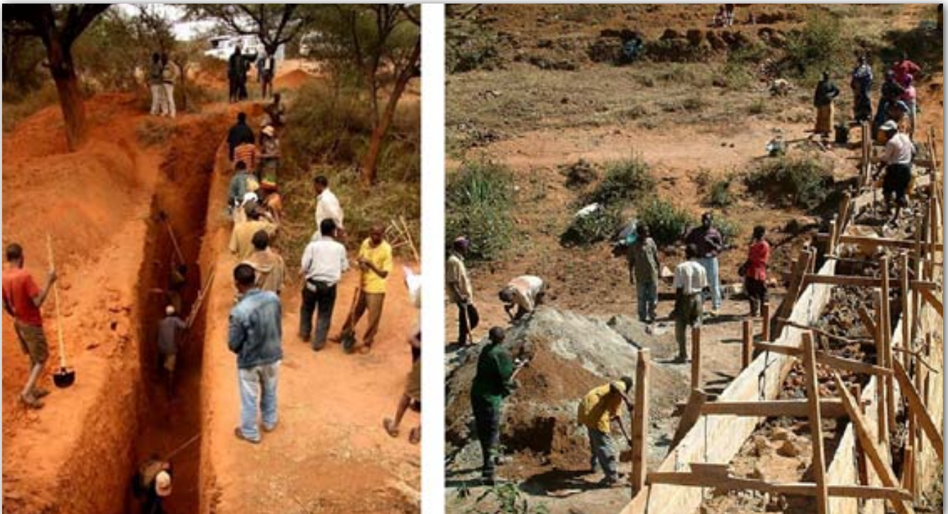
Fig 13.3 A typical layout & construction of sediment storage dam (SS dam) in arid & semi-arid areas
