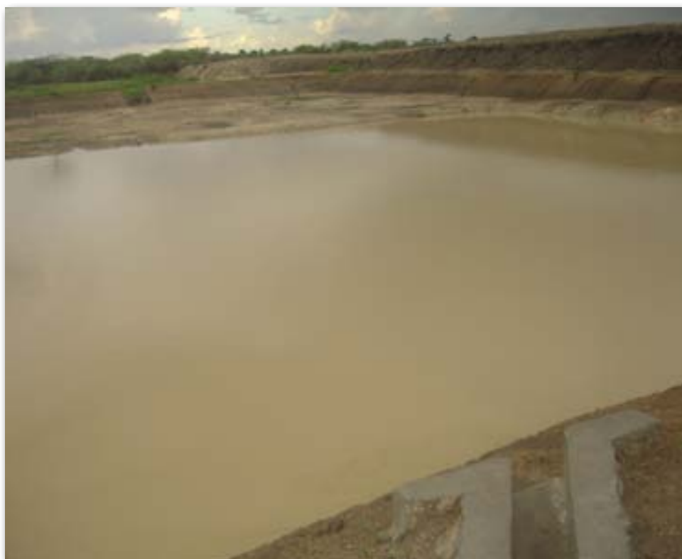
Fig 5.5 Shallow depth and wide storage areas lead to more evaporation losses (Napak)
