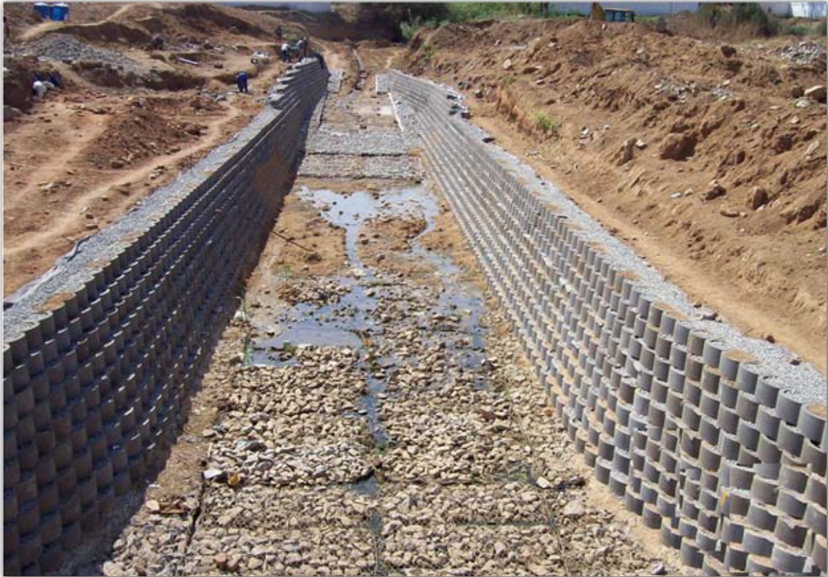
Fig 10.5: River bank erosion control is effective with retaining walls
