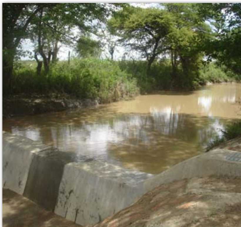
Fig 13.1 A typical sediment storage dam (Kotido)
