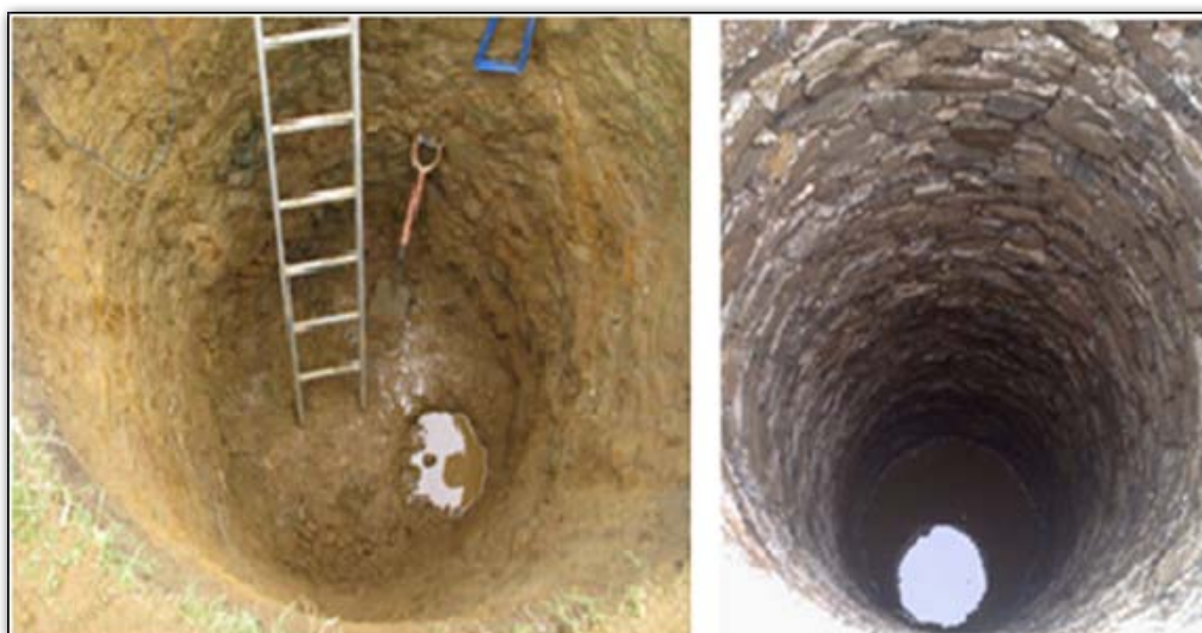
Fig 15.5: Manual hand dug well construction
