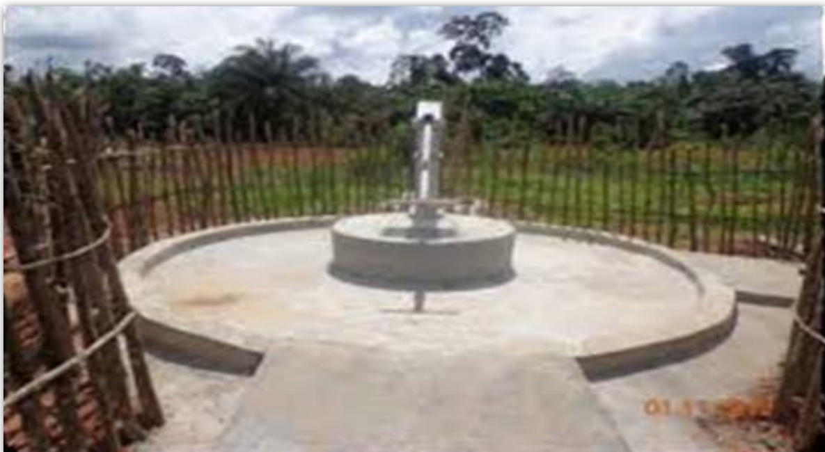
Fig 15.6: Shallow well with proper area drainage system
