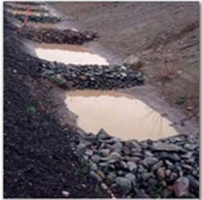
Fig 2.9 Impacts of gully check dams
